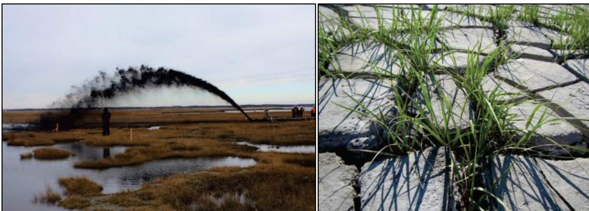
Figure 1. Thin Layer Placement (TLP) of sediment in marsh environments (left) are designed to increase marsh elevation and prevent subsidence, while allowing vegetation to recover (right). Photo credits: Tim Welp (left) and Christine VanZomerem (right).
